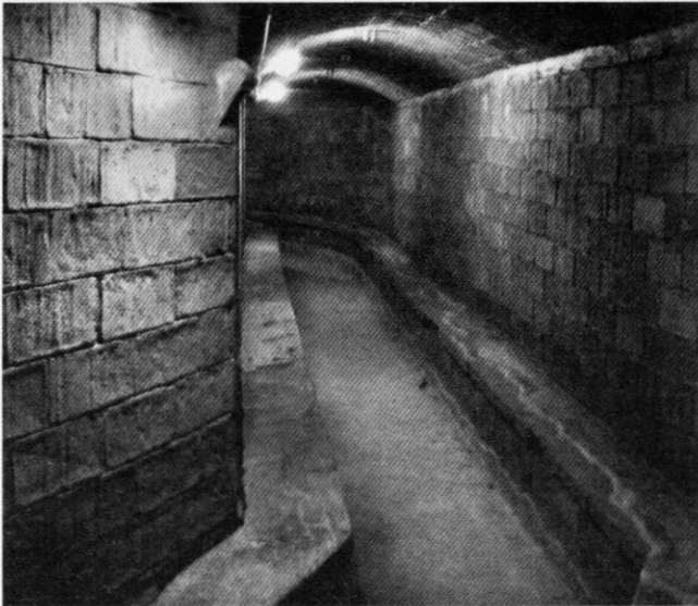
The shelter tunnels beneath Plaça del Diamant.
